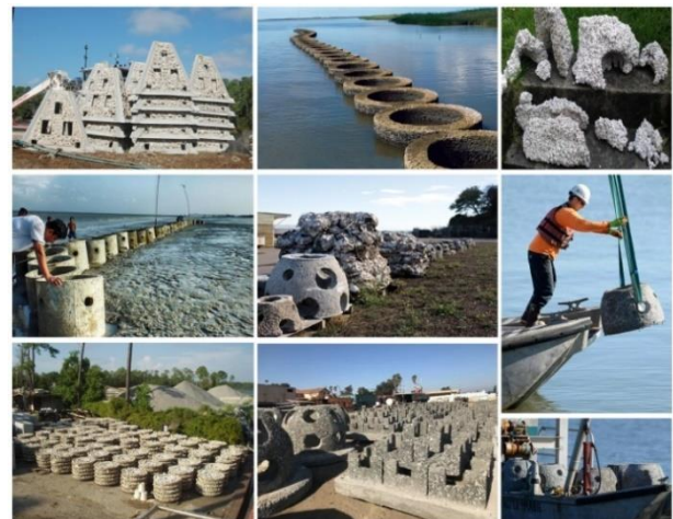
Figure 5. Artificial oyster reefs for oyster and herring populations, for shoreline protection and erosion control, for reducing wave action and promoting the establishment of plant and animal life in the vulnerable area
